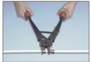
Pressfitting the joint using the hand-held pliers
