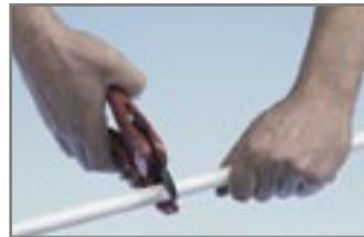
Cutting the TECEflex pipe using plastic cutters
