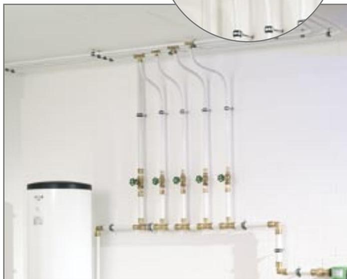
TECEflex sanitary installations make it possible to save costs and time when using this simplified connection and installation technology (see detail)
